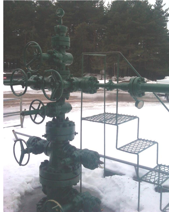
CO 2 Injection Well at Host Site
