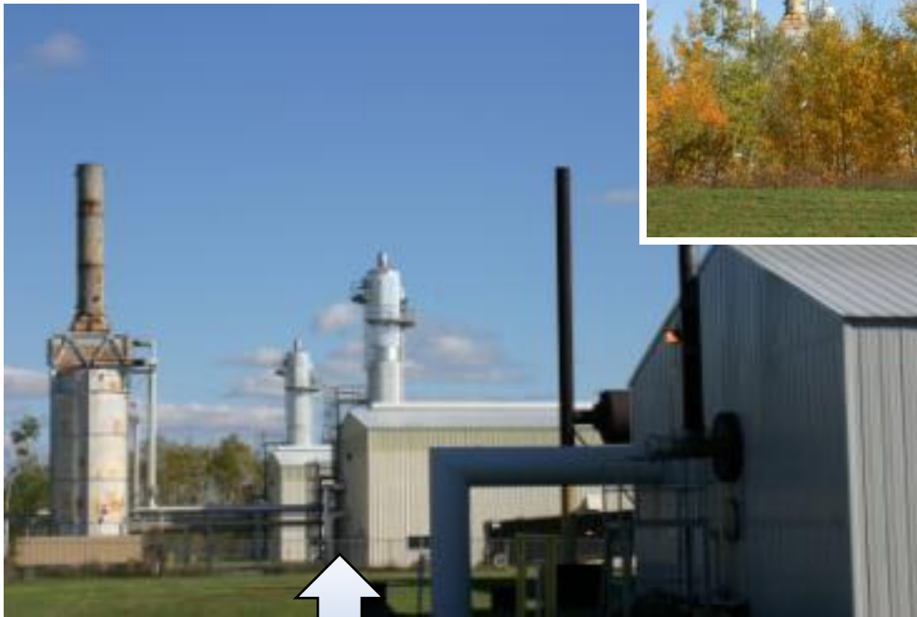
Gas Processing Plants
